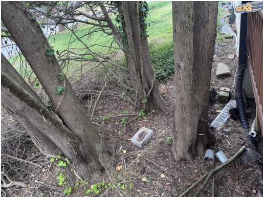
Leyland cypress trunks packed inches from the house and deck structure.
