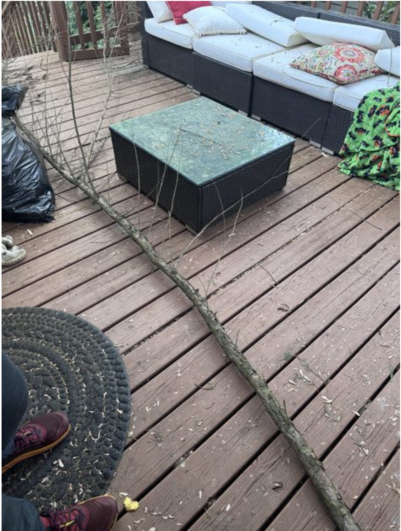
EXHIBIT E — Photo 10 of 11: Fallen branches and debris from the Leyland Cypress on the occupied deck surface. Active and ongoing fall hazard: branches and debris have already landed on the deck below. Consistent with the arborist's documented finding of 'dead trees in immediate danger of falling.'
